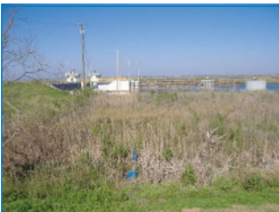
Bayou Terrebonne Water Control Structure
