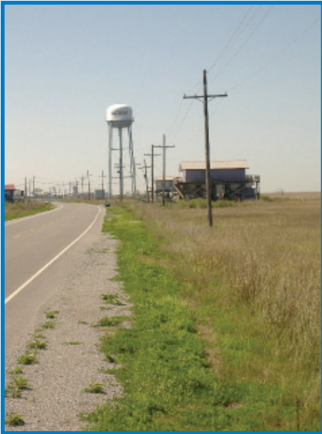
Consolidated Water Works in Terrebonne Parish, Louisiana
