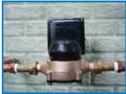
ORION® Meter Installation
