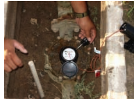
Installing the RTR®
