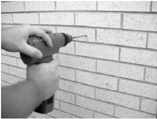
Drill Two Holes
