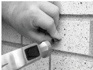
Place an Anchor in Each Hole
