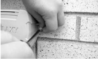
Screw in Transmitter
